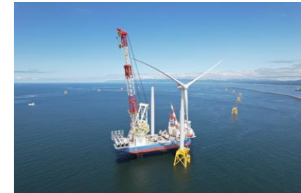
<Turbine Generator Installation>
